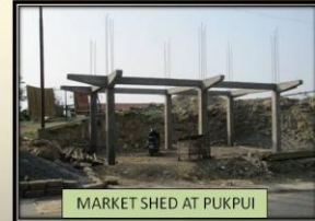
MARKET SHED AT PUKPUI
