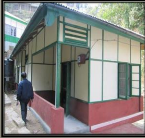
SUB-CENTER AT ELECTRIC VENG, LUNGLEI
